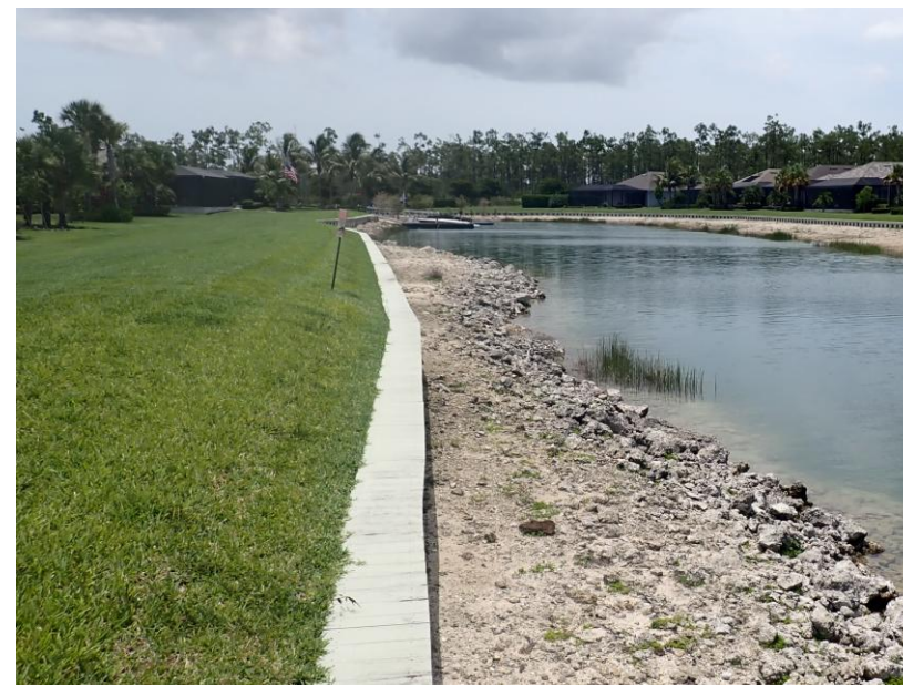
Existing Conditions (Narrow Shelf)
