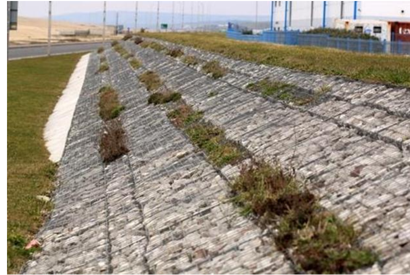
Metal Mattresses – vegetation can be installed
