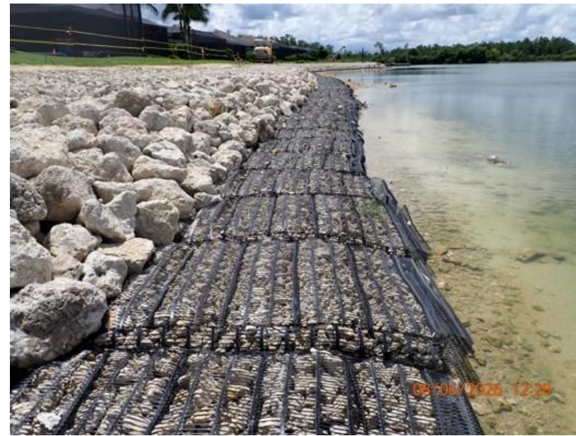
Rock Revetment with Marine Mattresses and Rock Apron
