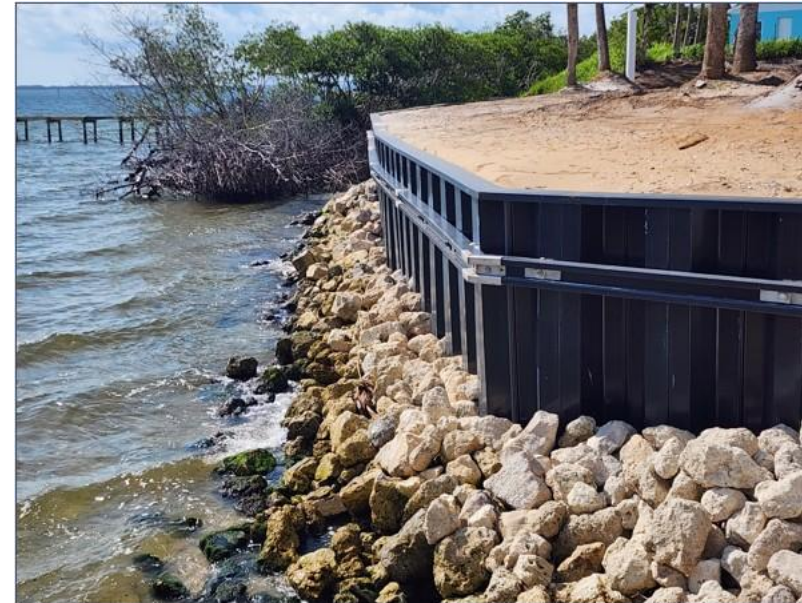
Retaining Wall with Toe Stones
