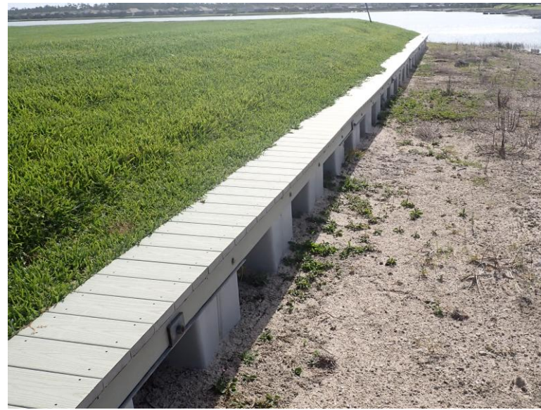
Retaining wall “intact and plumb”
