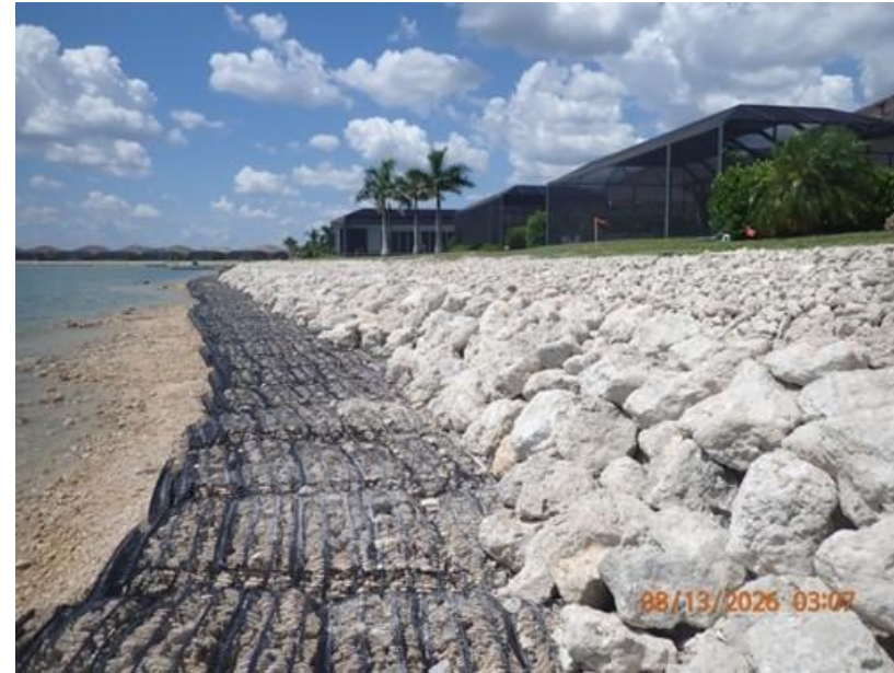
Rock Revetment with Marine Mattresses
