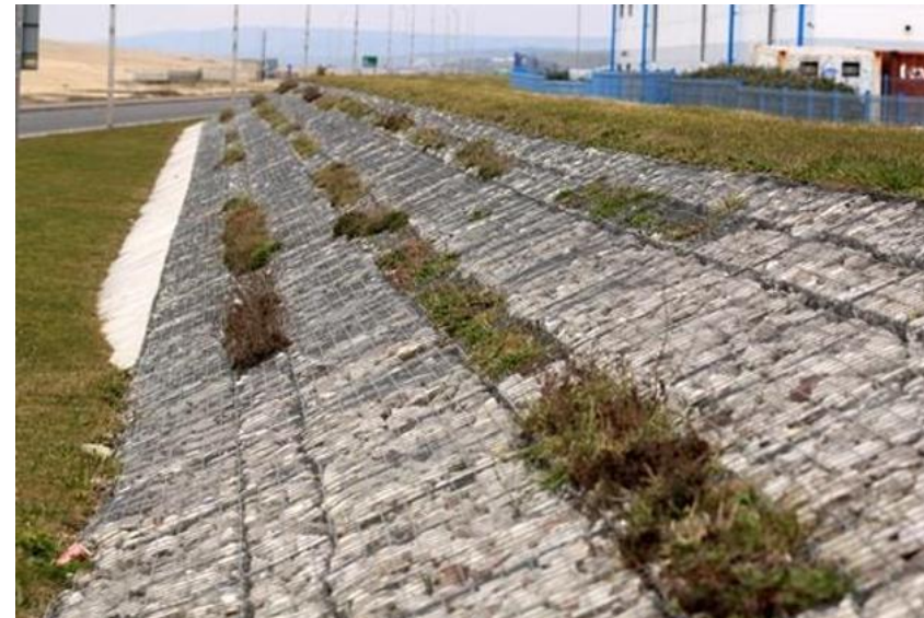
Metal Mattresses - vegetation can be installed
