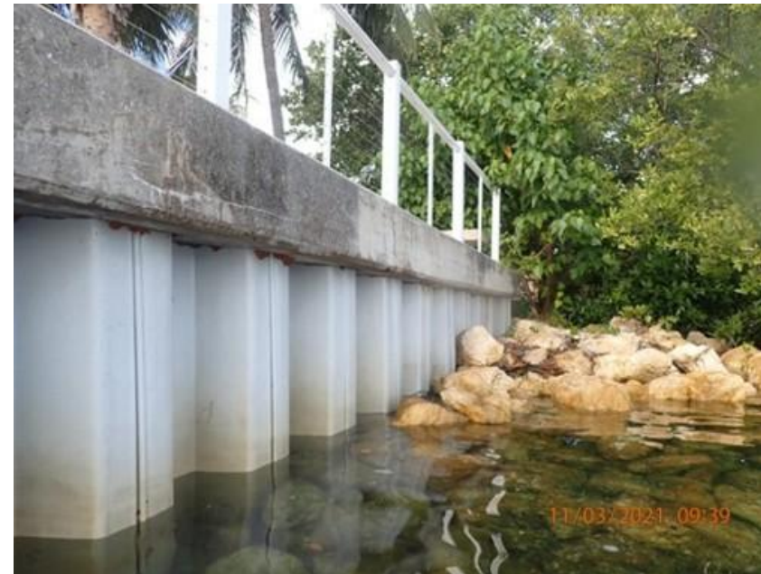
Vinyl Retaining Wall
