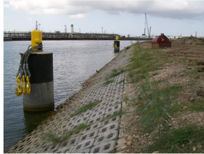
Open-Celled ACBs - vegetation can be installed
