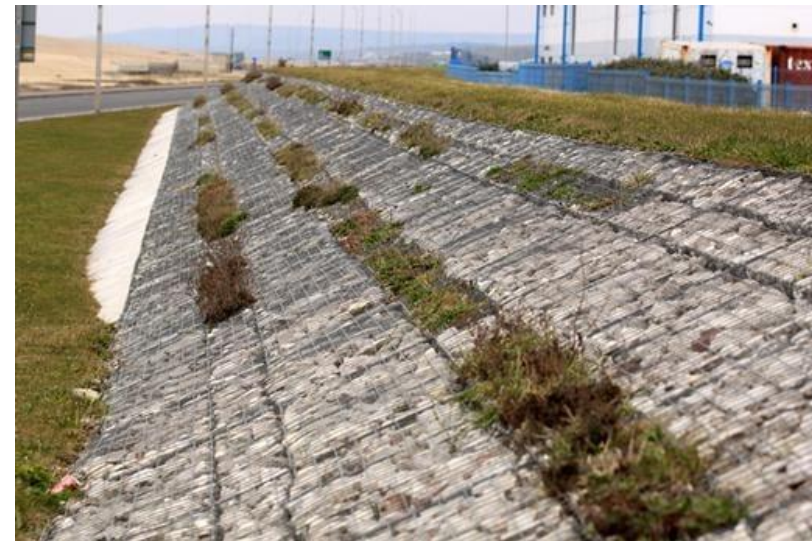
Metal Mattresses – Vegetation can be Incorporated
