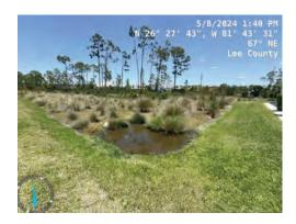
Recommendations: The observed conditions appear to be in accordance with the permitted design and no actions are recommended at this time. If desired, rip-rap may be added (generally 6" to 8" in diameter – typical size may vary) in the area immediately by water for aesthetic purposes.
