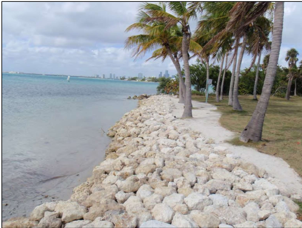
Photo 15. Limestone revetment.
