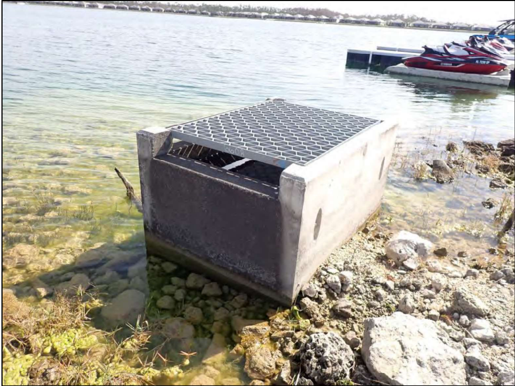
Photo 8. Lake level control weir.
