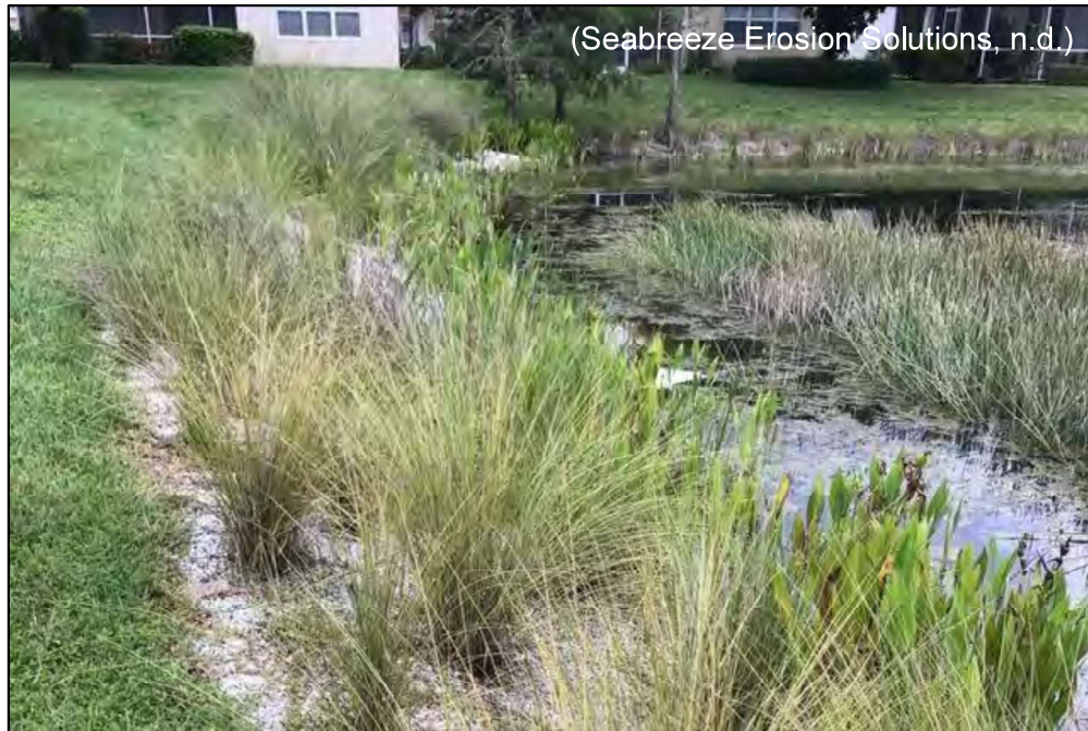
Photo 16. Living shoreline without rock breakwater.
