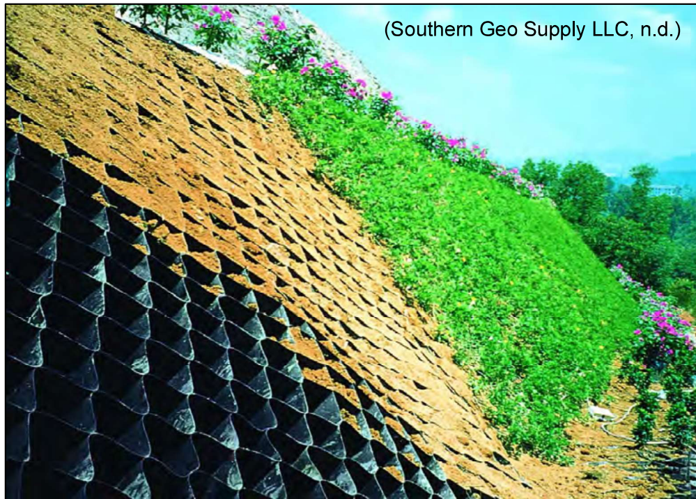
Photo 11. Geocells with vegetation.
