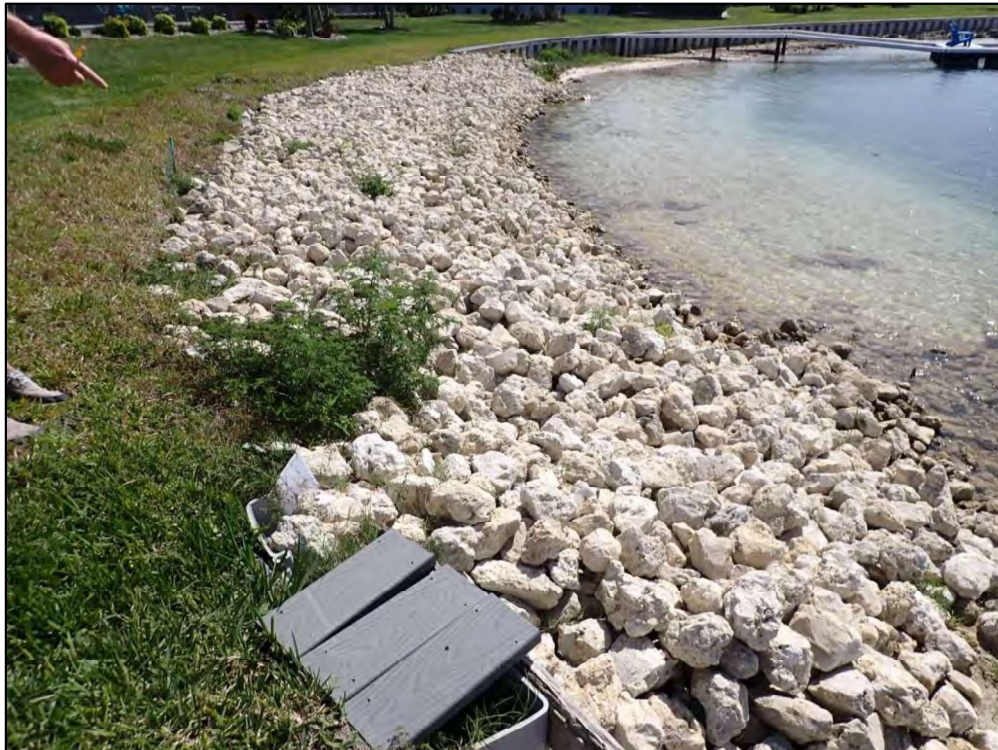
Photo 1. Seawall removed/encapsulated with riprap.
