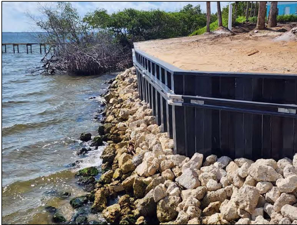
Photo 14. FRP retaining wall with toe riprap for scour protection.
