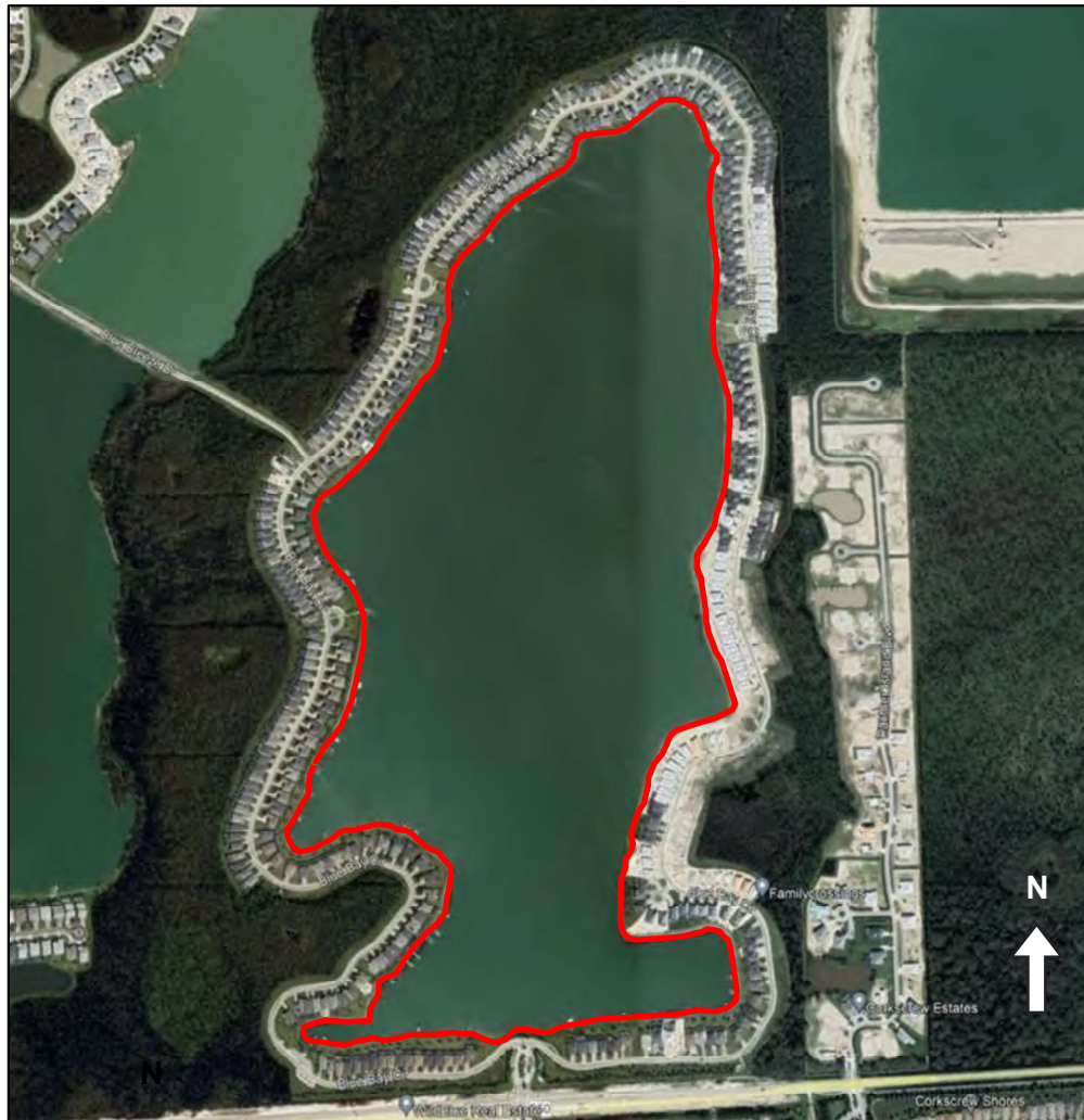
Figure 2. Project site, red line indicating a hardened shoreline structure.
