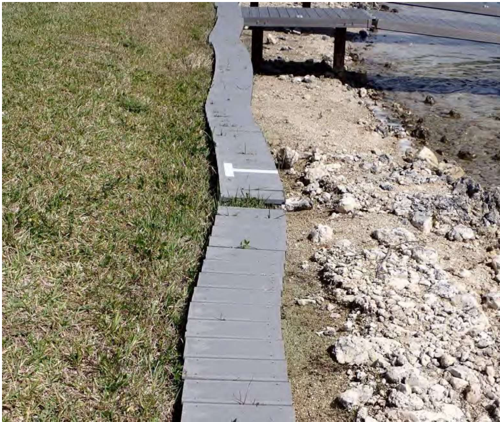
Photo 4. Typical central retaining wall.
