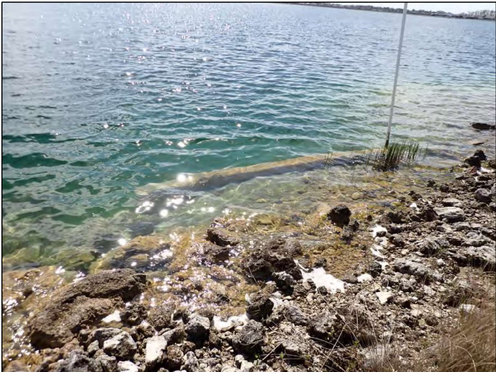
Photo 9. Submerged stormwater outfall headwall.
