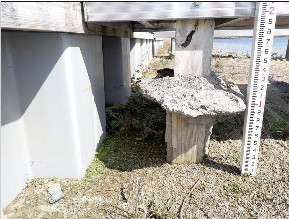
Photo 6. Sediment erosion on a dock piling.
