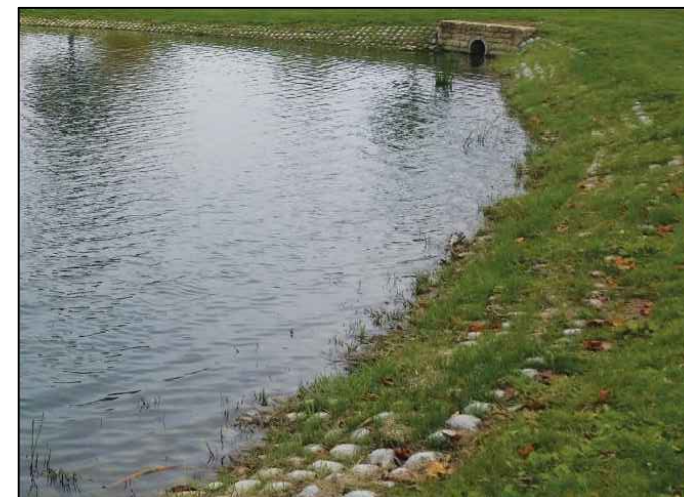
TYPICAL EROSION CONTROL MAT
