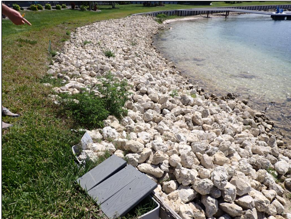
Photo 1. Seawall removed/encapsulated with riprap.
