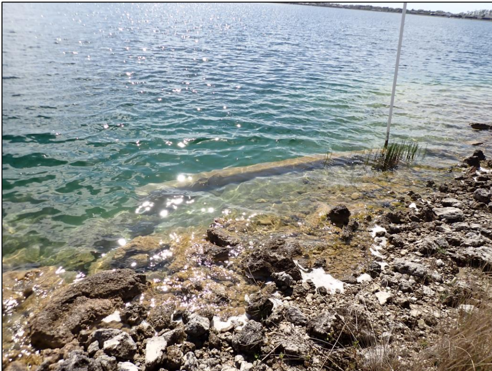
Photo 9. Submerged stormwater outfall headwall.
