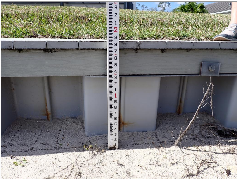
Photo 3. Seawall exposed height of approximately 1.85 feet.
