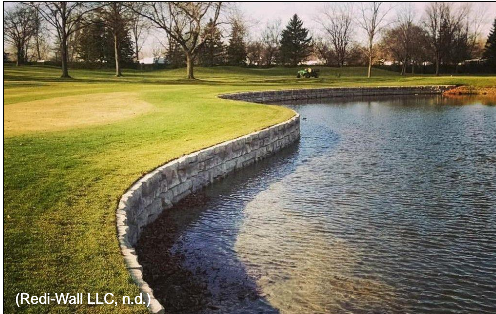
Photo 13. Modular block retaining wall.
