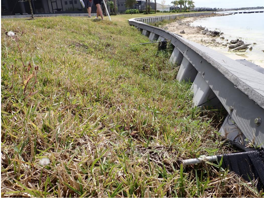
Photo 5. Severe waterward rotation and wall failure.
