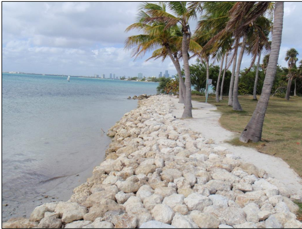
Photo 15. Limestone revetment.
